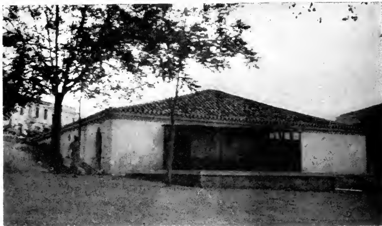
ANOTHER STORAGE RESERVOIR AT ATHENS ON THE HADRIAN AQUEDUCT
